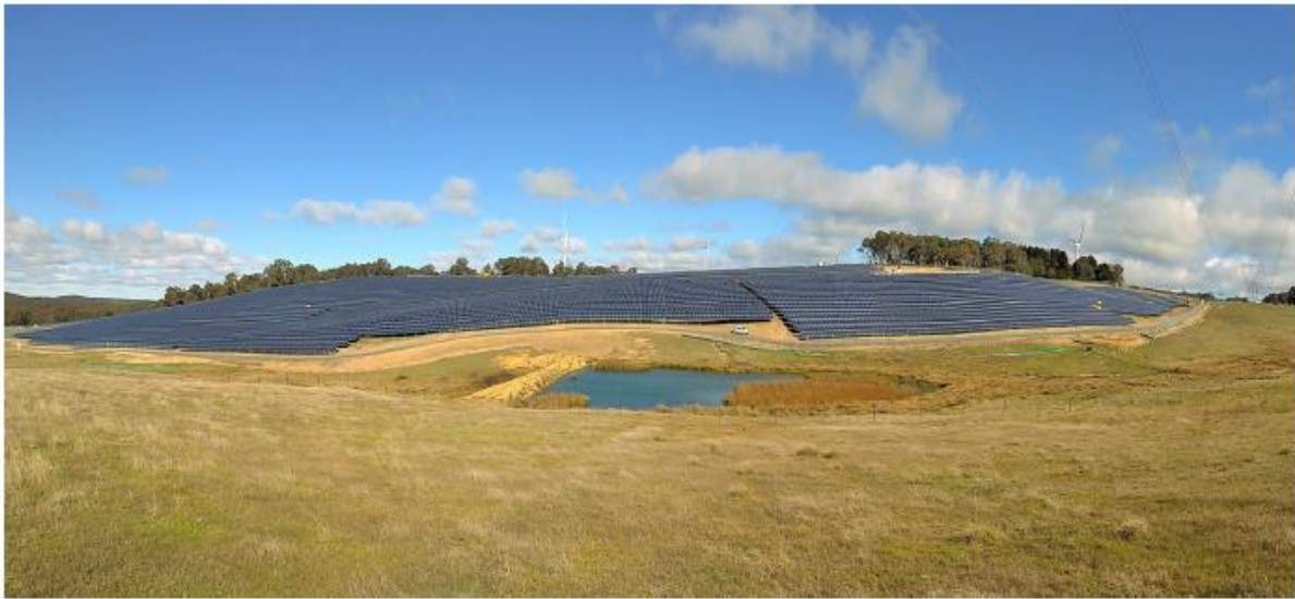
Current Construction Photo
