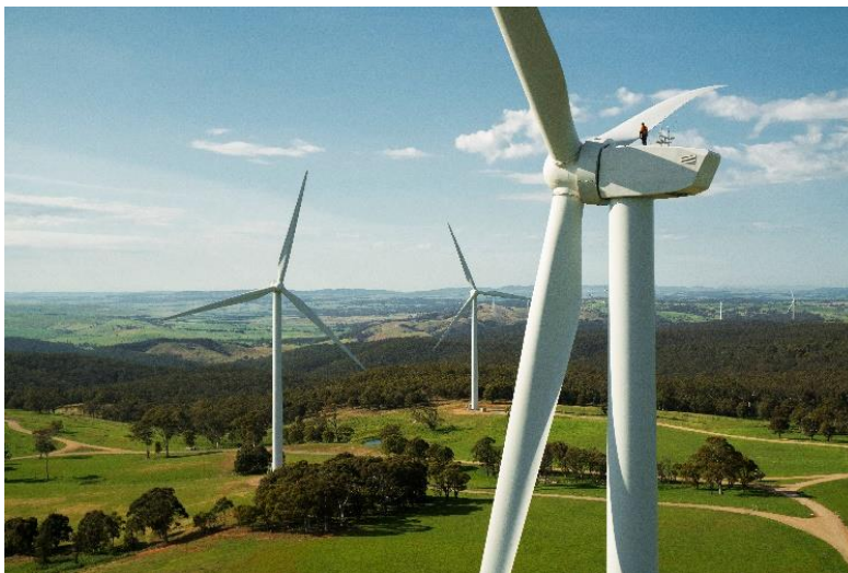
Image 1: Gullen Range Wind Farm (Photo: NGRWF)
